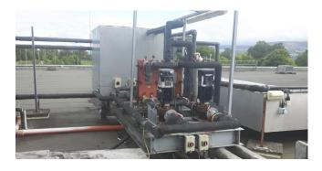
The manufacturing site at Clonmel needs a constant water temperature of 14 degrees on the lasers or they cut out and production halts. The existing heat exchange unit was no longer functioning efficiently, so a new solution was needed, and quickly. The team at Campion had 3 months to design, fabricate, test a new heat exchange unit with one day installation and commissioning to prevent any down time in manufacturing.
